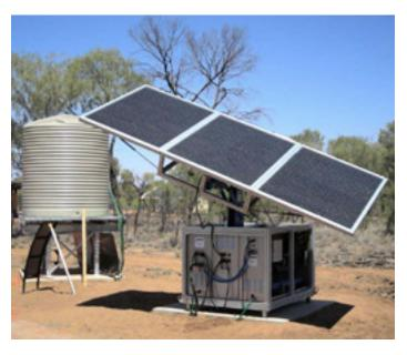
The €40,000 (\$60,000) RO system pictured above was installed at Alice Springs, Australia and operated on groundwater with a 15,000 mg/L TDS. It produced 5,000 L/d (1,320 GPD) of drinking water at a cost of approximately  $€3.00/m^3$  (\$4.44/m³; \$16.81/kgal), based on a 5-year amortization.
